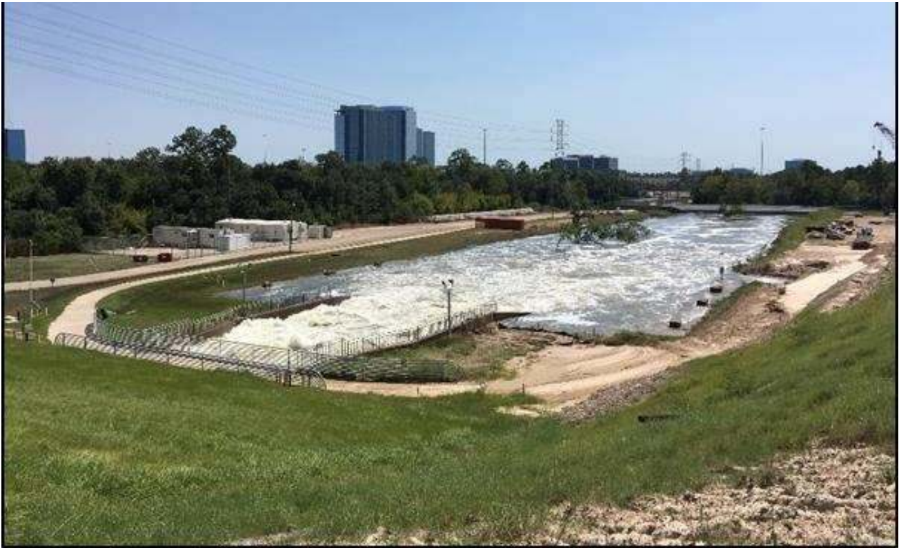
Figure 5. Addicks outlet releasing \sim 170 \text{ m}^3/\text{s} ( \sim 6000 \text{ cfs} ) (September 9, 2017, 29.79026^\circ \text{ N} , 95.62378^\circ \text{ W} ).
