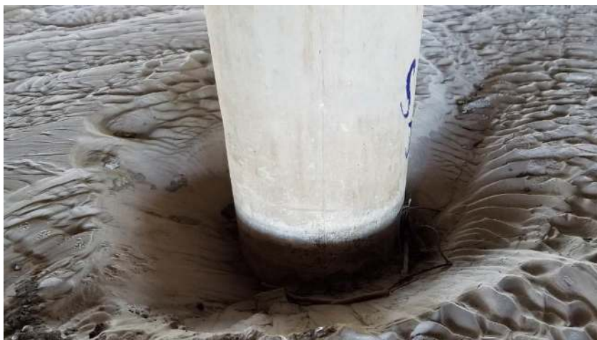
Figure 40. Scour around columns on San Jacinto Banks (sandy soil). The scour hole was approximately 2.4 m (8 ft) across and 0.6 m (2 ft) deep (September 11, 2017, Time 10:59 CDT, 30.243364°N, 95.46452°W).
