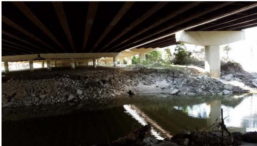
Figure 39. Riprap along south bank of San Jacinto River (September 11, 2017, Time 10:56 CDT, 30.24574° N, 95.45761° W).
