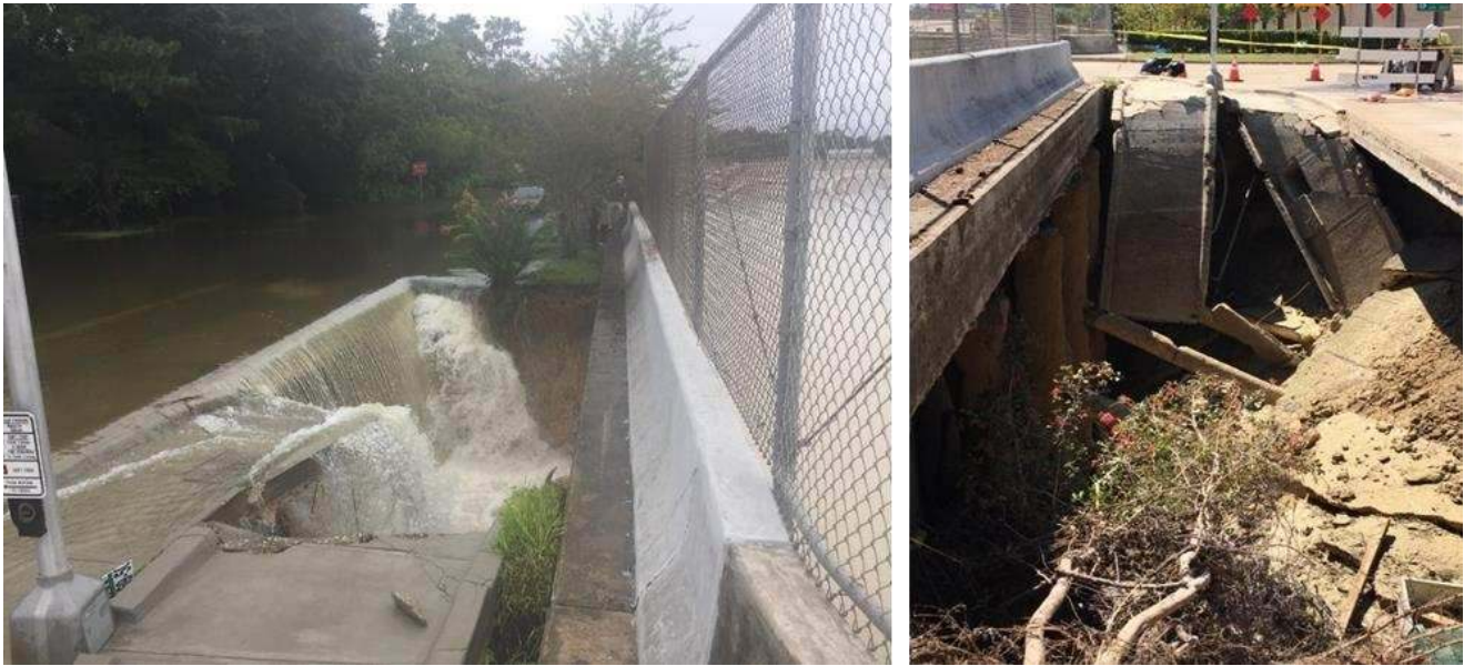
Figure 32. Damage of the walkway slab on Beltway 8 (left photo courtesy Brian Klein, a resident in the area, August 27, 2017, and right photo courtesy of a construction worker on site, 29.76735° N, 95.56219° W).
