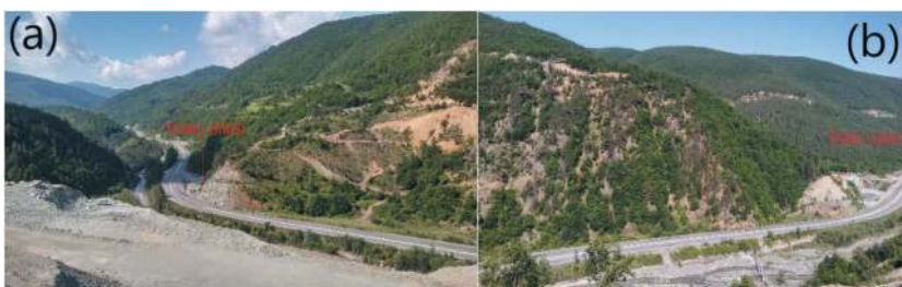
Figure 1. General field photographs of the diversion tunnel project site: (a) view of the tunnel inlet area; (b) view of the tunnel outlet area.
