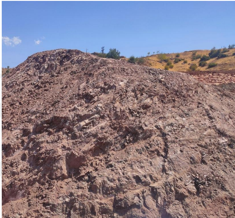
Figure 4.80. Photo showing the highly fractured ophiolitic mélange matrix and residual soil mantle
