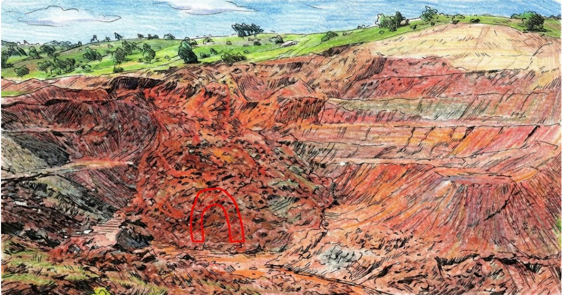
Figure 4.56. Illustration of the diversion tunnel exit portal closure and associated slope failure
